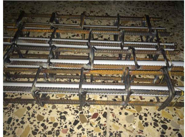
(b) Preparing the reinforcement cage
