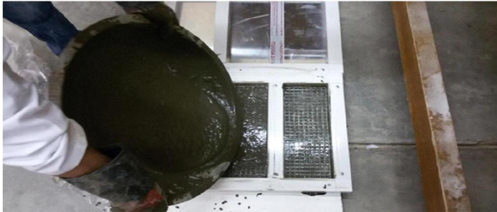
**Figure (1):** Casting of the ferrocement panels.
