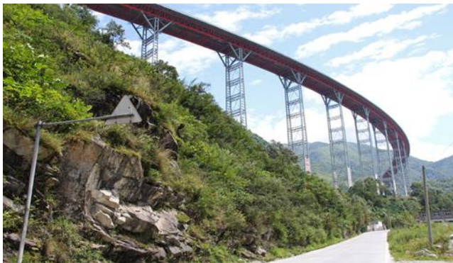
Figure 1: Ganhaizi Bridge, China.
