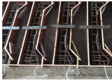
c- Installing thermocouples to the steel bar
